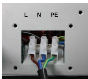
Fig. 8 AC terminals under AC terminals cover
